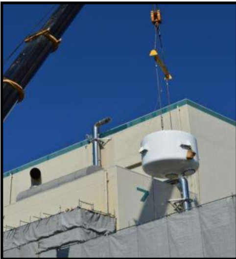
TEPCO's Kashiwazaki-Kariwa Unit 7. AgX filter to be brought in (Kashiwazaki Kariwa Nuclear Power Station Unit 7)
